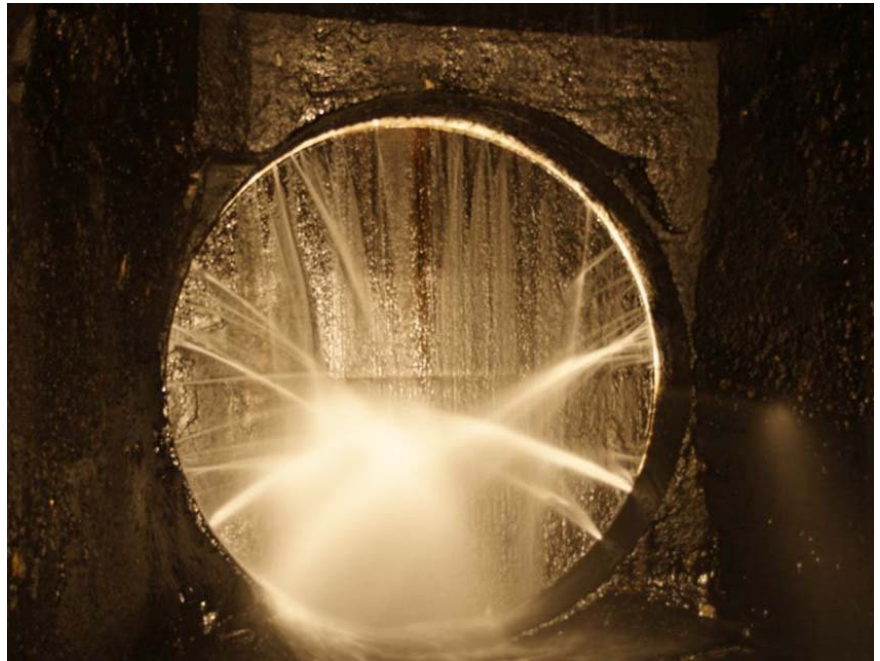
Maintenance gate downstream access when the gate is closed. Installed in 1909. Gate sluice failed and replaced in 1954.
