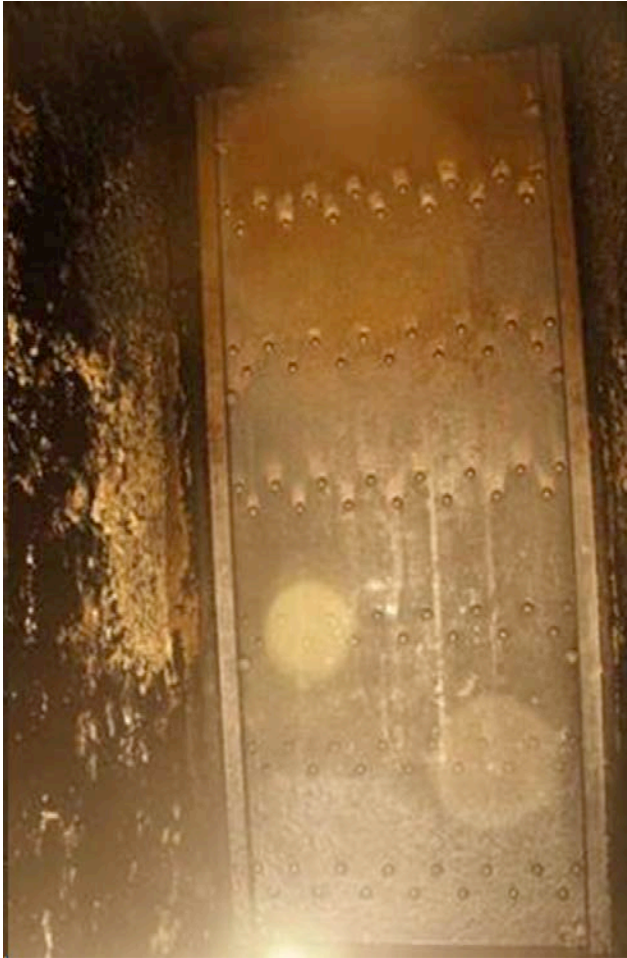
Operating gate (one of two) installed in 1911 does not meet current safety standards.
