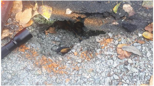
The sinkhole looks minor at this point, but it does show there has been a significant amount of granular material migration. The sinkhole will continue to worsen over time. The municipal watermain is located within the failure zone, and could potentially cause a failure of the watermain.
