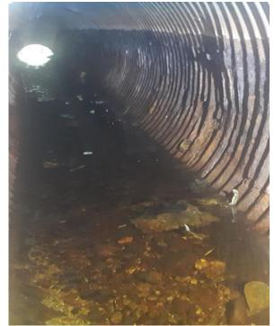
There is a significant collaspe on the northern end of the culvert. This is restricting storm flows within the culvert. The restriction will cause surcharging during a storm event, which can potentially cause damage to property and Village infrastructure. The collaspe has also caused a sinkhole to develop on Strong Road.
