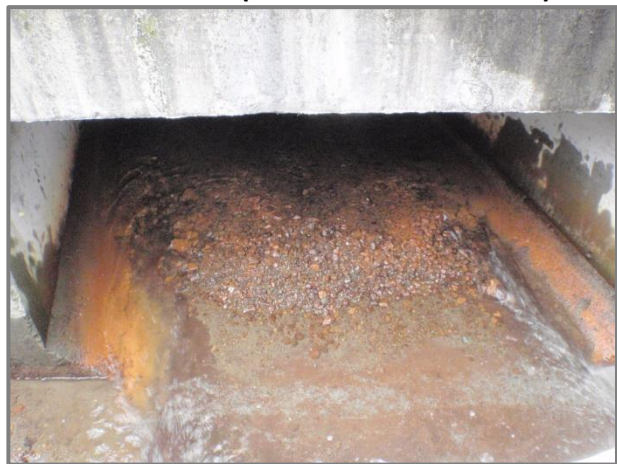
Inlet Picture (Weir Not Installed Yet)
