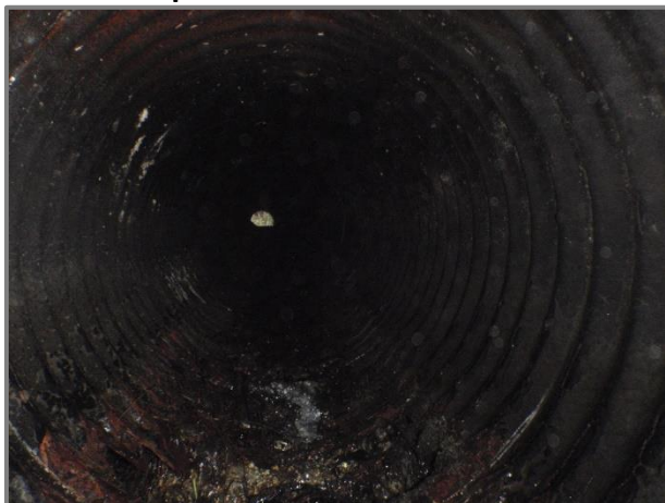
Upstream Conduit Picture
