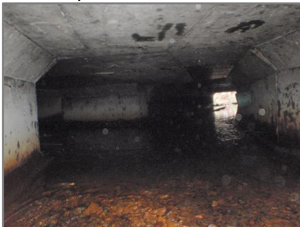
Upstream Conduit Picture
