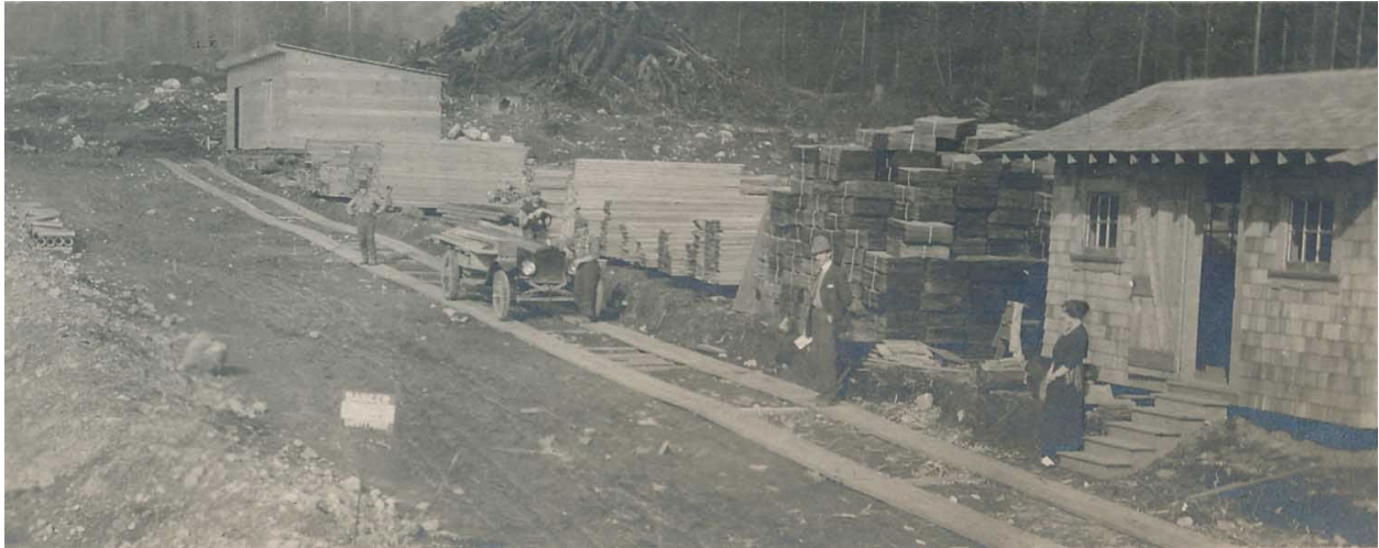
Figure 5. Construction of houses at what became the Ioco Townsite, ca. 1921. [POMO Port Moody Museum, 2023 https://www.pomo.museum/ioco-chapter-4 ].
