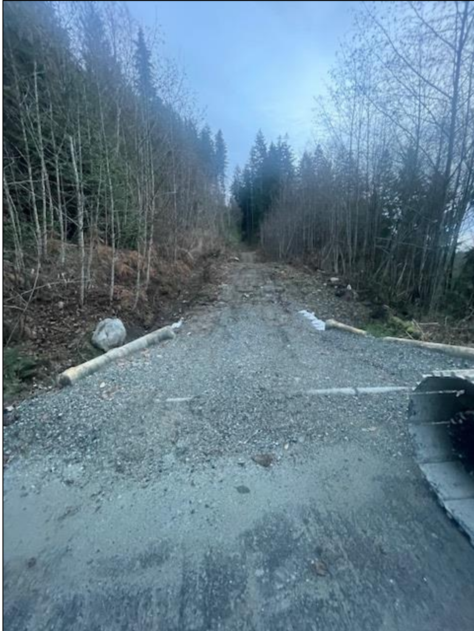
Photo 19: Access road at south extent of North Charlotte Drive (December 13, 2023)
