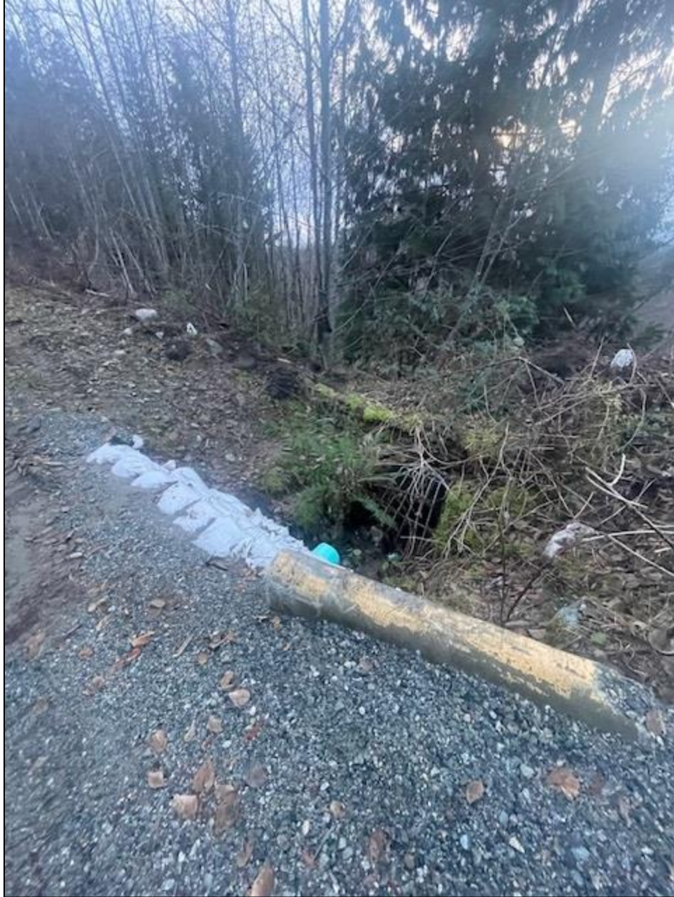
Photo 20: Minor Drainage System #2, stormwater drainage pipe intake at west side of North Charlotte Drive extension (December 13, 2023)
