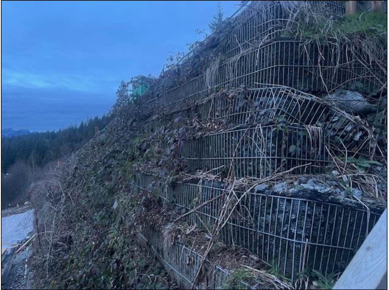
Photo 29: MSE Retaining wall along west/downslope side of Ridge Mountain Drive (December 13, 2023)
