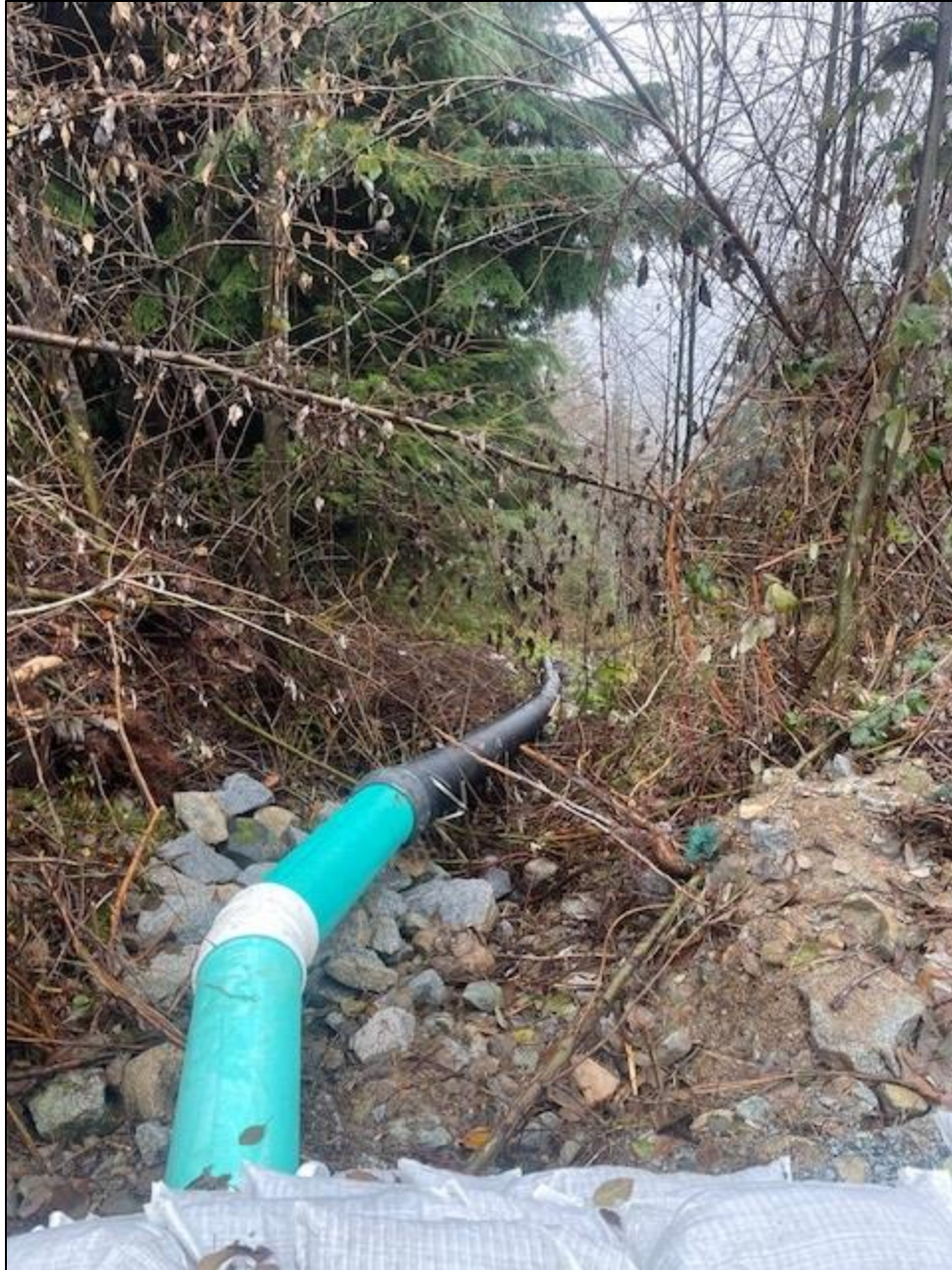
Photo 8: Minor Drainage System # 2, stormwater drainage pipe at south extent of asphalt paved Ridge Mountain Drive, collecting drainage from the swale shown in Photo 7, looking downslope/west (December 11, 2023)
