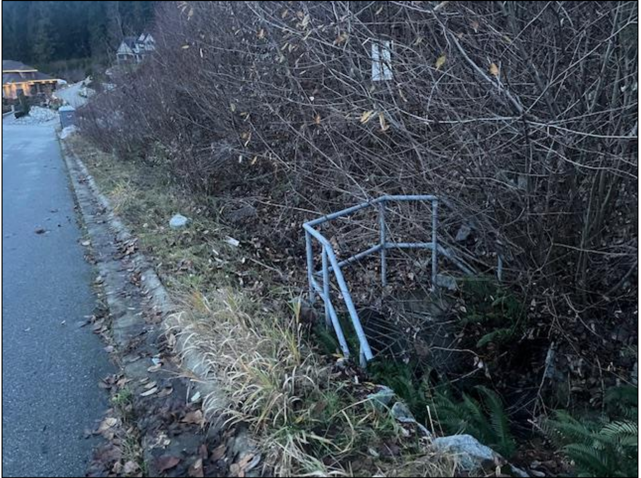
Photo 27: Minor Drainage System #1 upslope of culvert at Ridge Mountain Drive (December 13, 2023)
