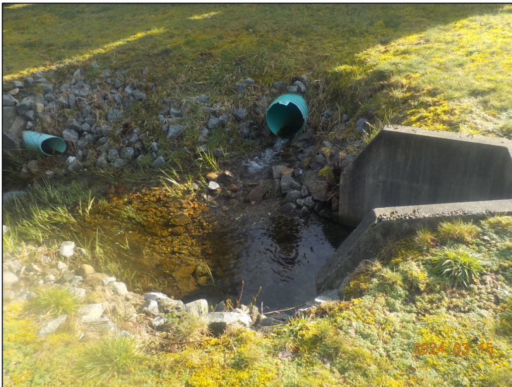
Photograph 15. View of Watercourse E (March 15, 2024).
