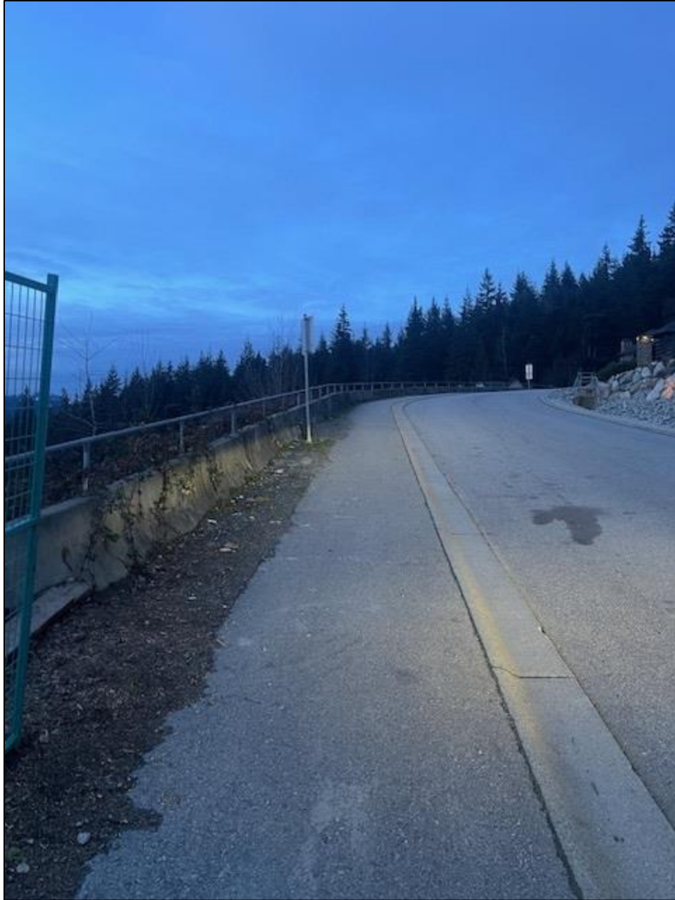
Photo 24: MSE Retaining wall along west/downslope side of North Charlotte Drive (December 13, 2023)
