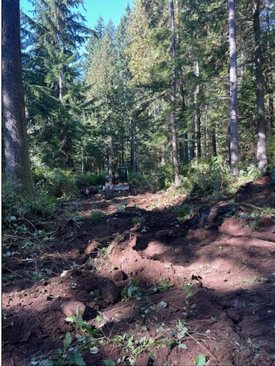
Photo 4: New access road from Ridge Mountain Drive extension (October 6, 2023)
