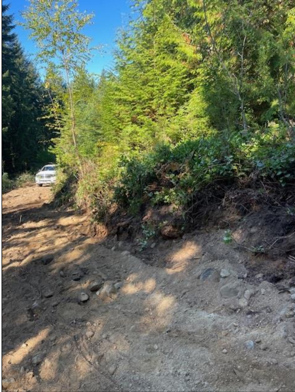
Photo 3: New/re-worked access road from Ridge Mountain Drive extension (October 6, 2023)
