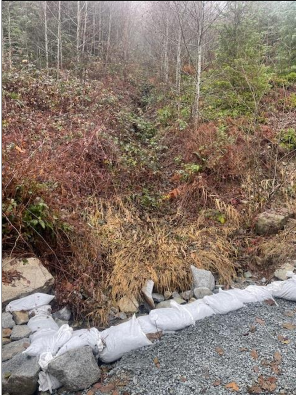
Photo 7: Minor Drainage System # 2, drainage swale at south extent of asphalt paved Ridge Mountain Drive, collecting drainage from the cross-slope swale within TREZ development area, looking upslope/east (December 11, 2023)
