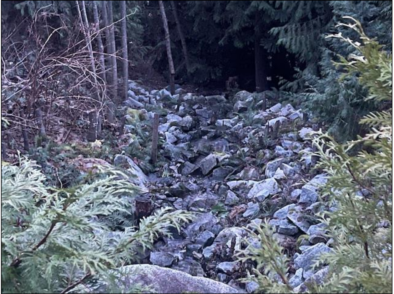
Photo 26: Minor Drainage System #1 downslope of culvert at Ridge Mountain Drive (December 13, 2023)
