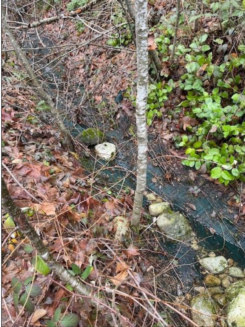
Photo 15: Cross-slope swale at southern portion of TREZ development (December 13, 2023)
