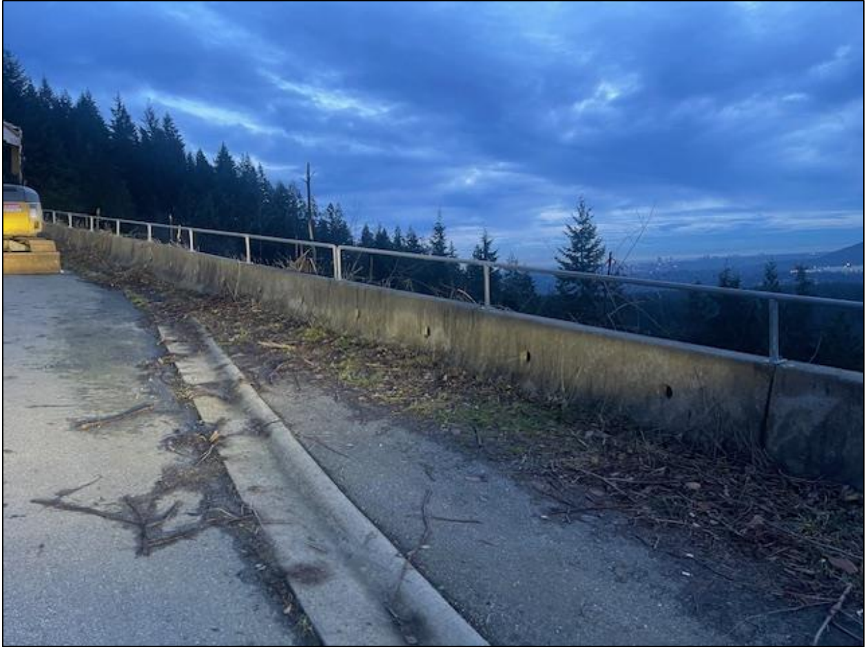
Photo 28: MSE Retaining wall along west/downslope side of Ridge Mountain Drive (December 13, 2023)
