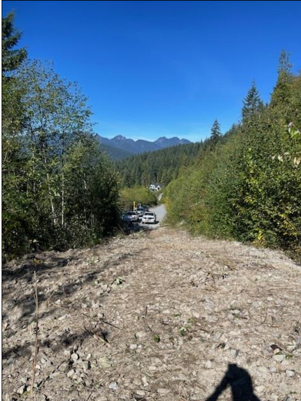
Photo 1: Existing access road extension from Ridge Mountain Drive, looking north (October 6, 2023)
