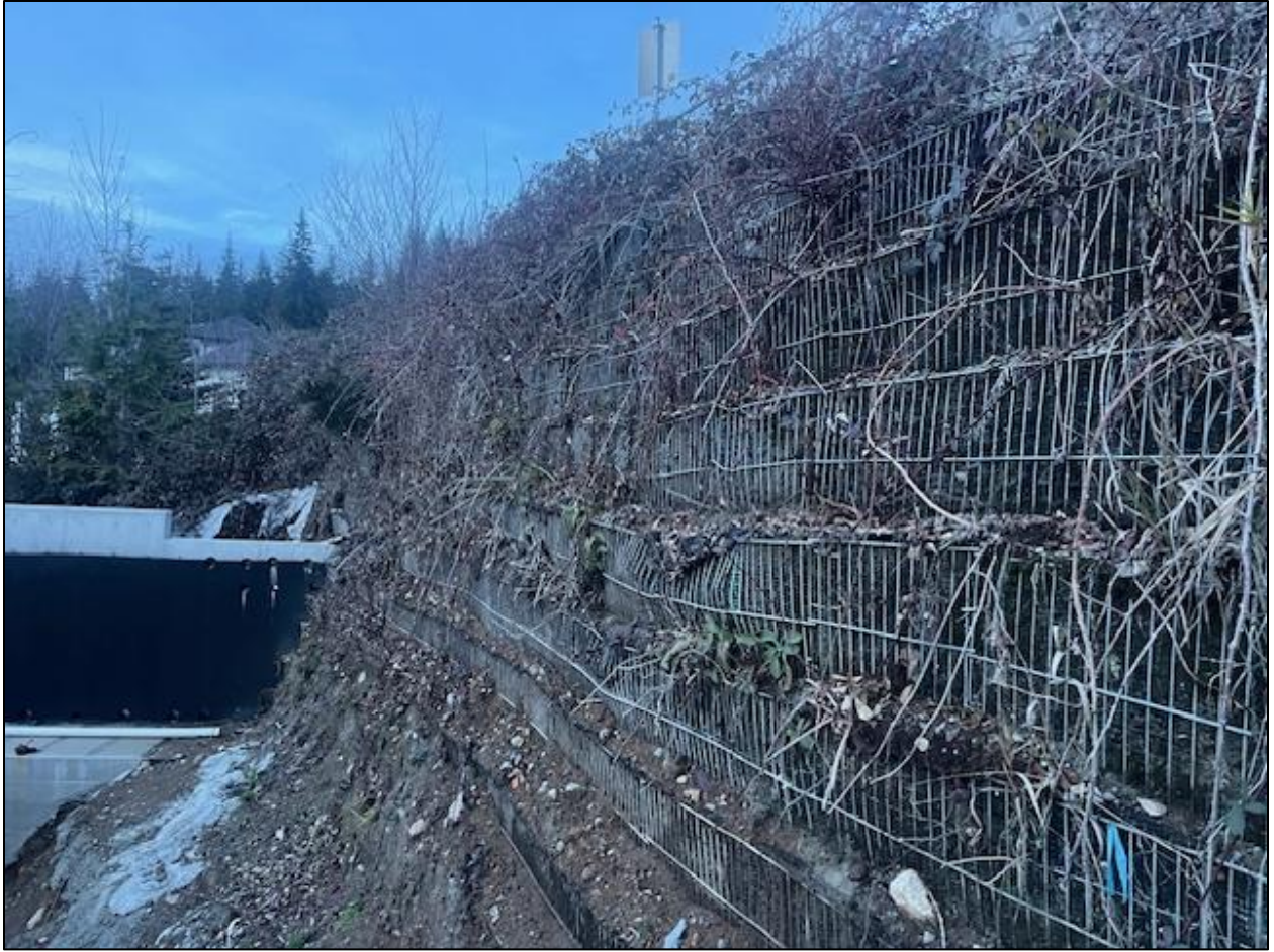
Photo 25: MSE Retaining wall along west/downslope side of North Charlotte Drive (December 13, 2023)
