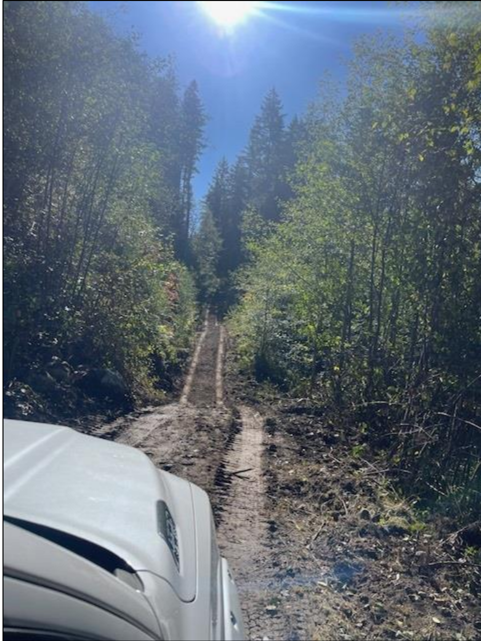
Photo 2: Existing access road extension from Ridge Mountain Drive, looking south (October 6, 2023)
