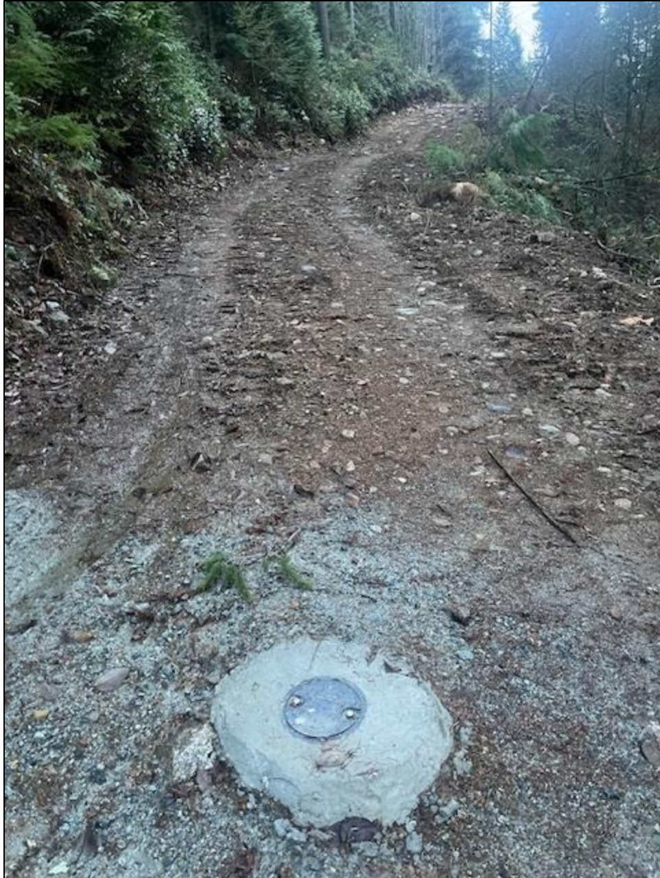
Photo 22: North Charlotte Drive extension and groundwater monitoring well (December 13, 2023)
