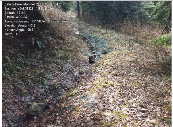
Photo 12 – Looking south and downstream at the unnamed drainage with the deactivated road on the west side and forest on the east side. View of man-made mesh trench for drainage (Feb 20, 2017).
