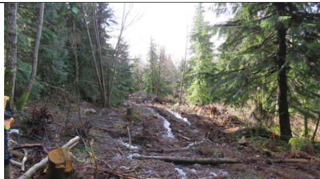
Photo 2. A road currently under construction within the RFVT (February 20, 2017).
