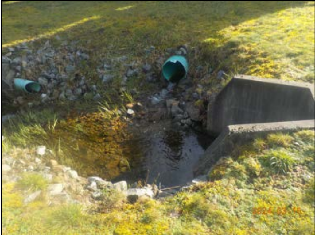
Photograph 15. View of Watercourse E (March 15, 2024).
