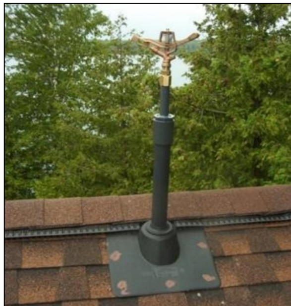
Figure 11. Examples of rooftop mounted sprinkler systems: temporary (left) and permanent (right)
