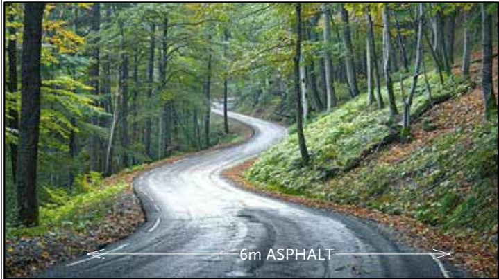
SECONDARY TRAIL 512m Proposed Secondary Trail (emergency access road) Paved, 6m wide, 15%max
