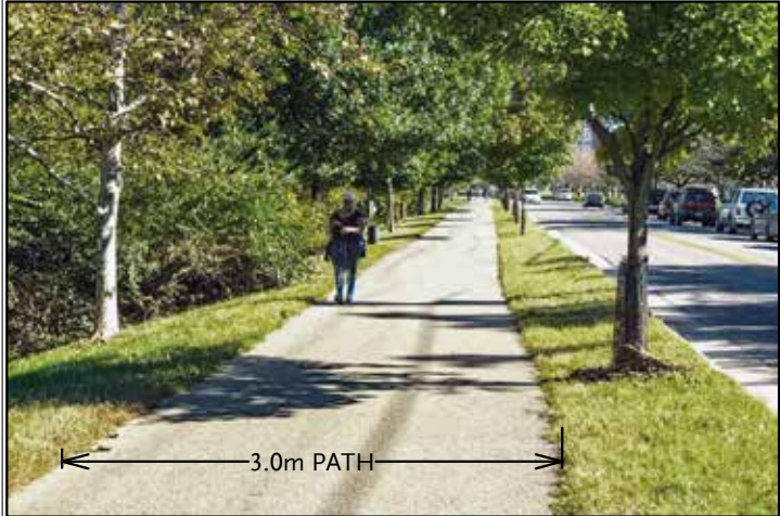
MULTI-USE PATH 2,561m Proposed Multi-Use Path 3.0m width, in R.O.W. (212m off-site @Wyndham)
